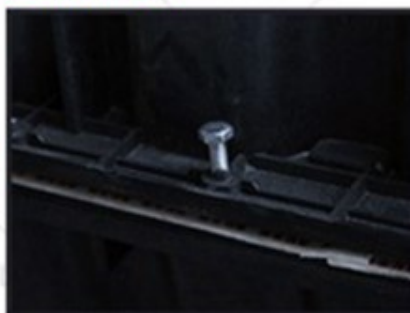
8. Sealed by bolts and nuts
