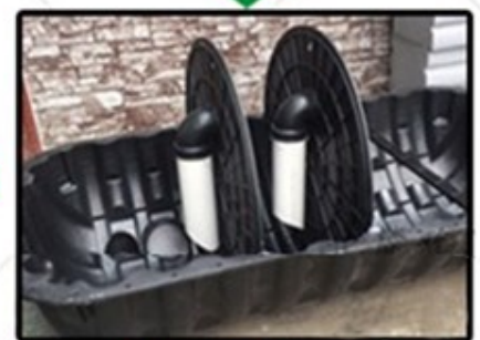
4. Install filter pipe
